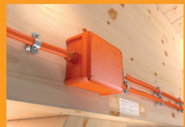
Mounting of the OBO FireBox on a wooden beam.
