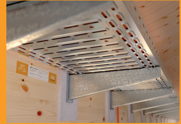
Bracket mounting on the side of the wooden beam with rear fire protection plate.
