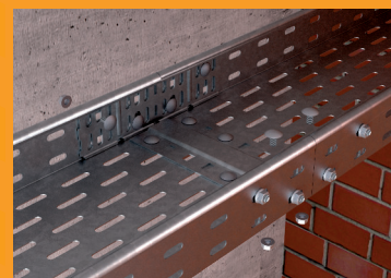
Fasten straight connectors and joint plate using truss-head bolts.
