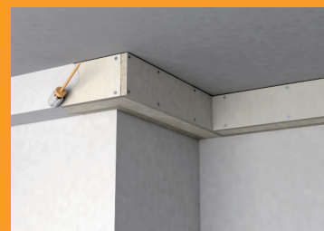
Closing surface treatment through painting or papering.
